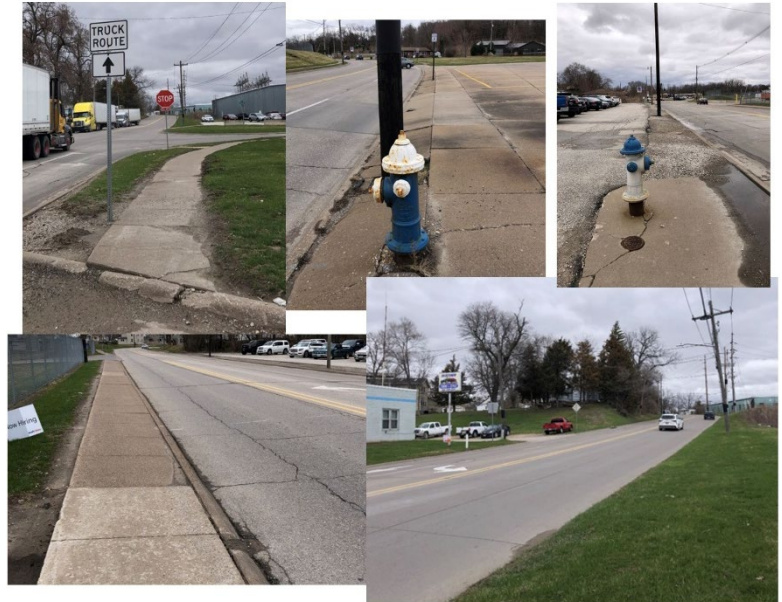
Figure 15: Sidewalks without a buffer from the roadway, curb cuts, adequate crosswalks, or that are altogether nonexistent discourage pedestrian and bicycle traffic along Isett Avenue.
