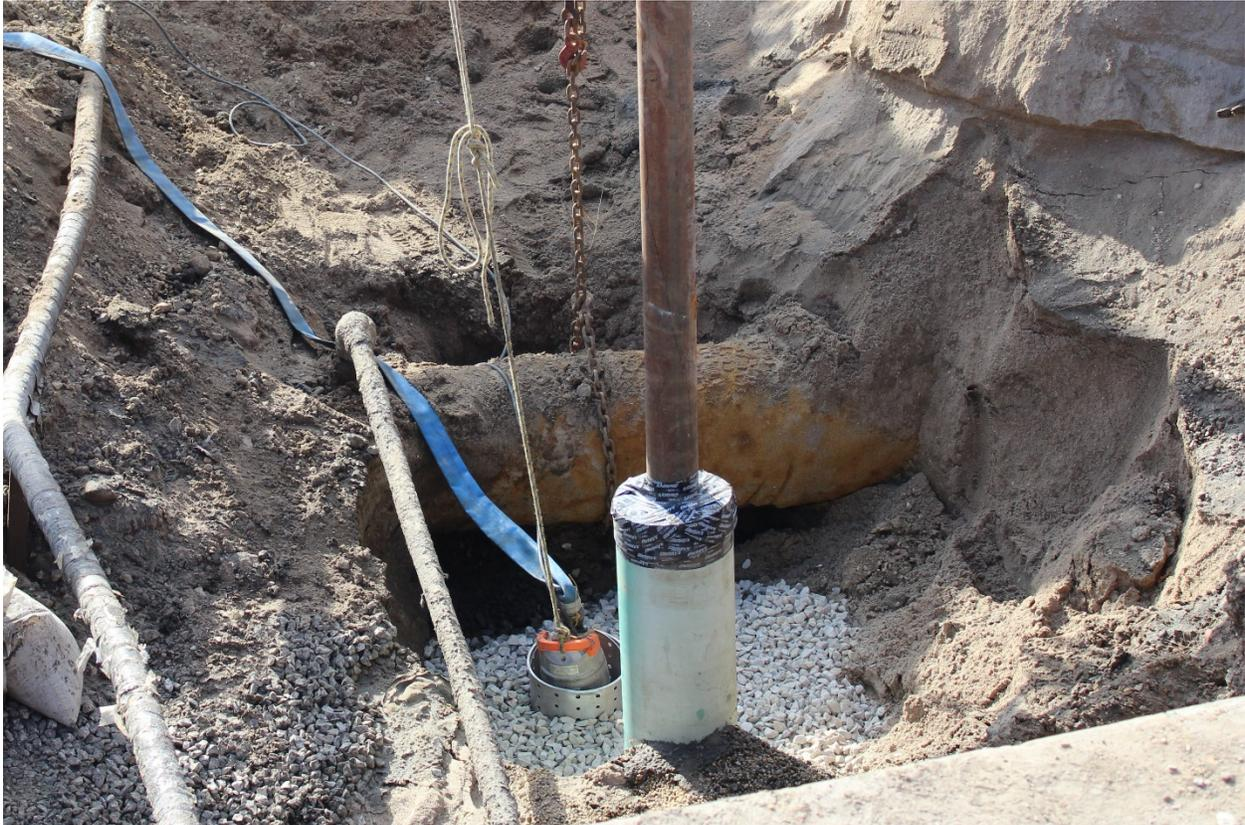
**The water main is exposed but the suspected culprit of the leak, the 30-inch force main, still lies unexposed. The 16-inch water line will have water stops placed on Wednesday to allow crews to continue digging down to the sewer line. The City suspects that the leak is coming from the force main but will not be certain until the line is exposed.**
