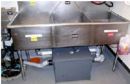
A trap is a small reservoir built into the wastewater piping a short distance from the grease producing area. Baffles in the reservoir retain the wastewater long enough for the grease to congeal and rise to the surface. The grease can then be removed and disposed properly. See *How Grease Traps and Interceptors Work* for a description of how the various components of grease traps function.
