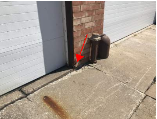
③ REPLACE CRACKED OR SPALLED BRICK
