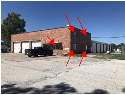
④ REPLACE SEALANT AROUND WINDOW
