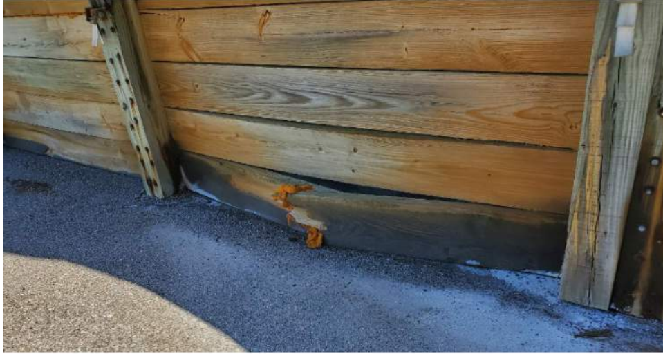
Figure 10. Out-Building 1 Broken Wall Plank
