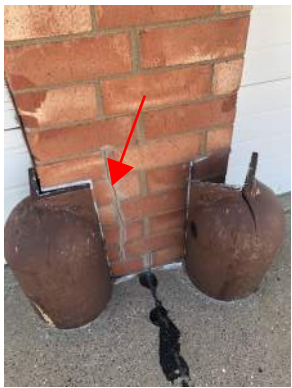
③ REPLACE CRACKED OR SPALLED BRICK
