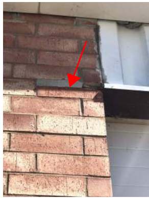
③ REPLACE CRACKED OR SPALLED BRICK
