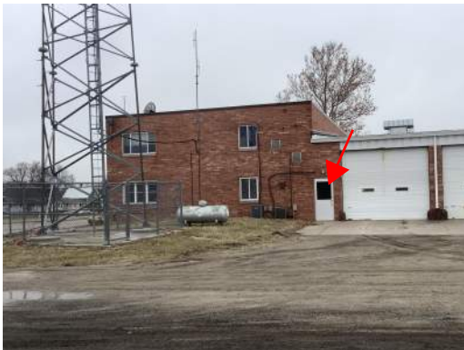
⑤ REPLACE SEALANT AROUND DOOR
