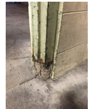
⑧ REPLACE RUSTED DOOR AND FRAME ASSEMBLY
