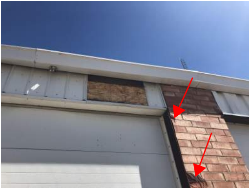
③ REPLACE CRACKED OR SPALLED BRICK
