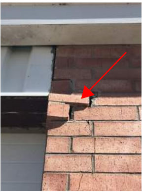
③ REPLACE CRACKED OR SPALLED BRICK
