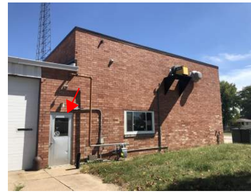
⑤ REPLACE SEALANT AROUND DOOR
