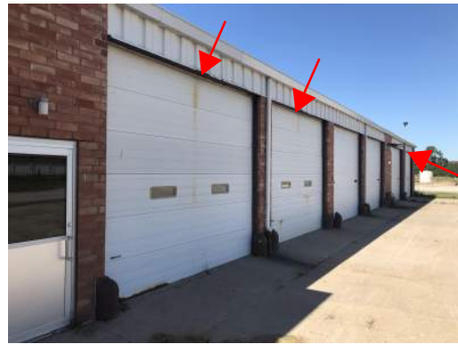
⑩ REPLACE RUSTED OVERHEAD SECTIONAL DOOR
