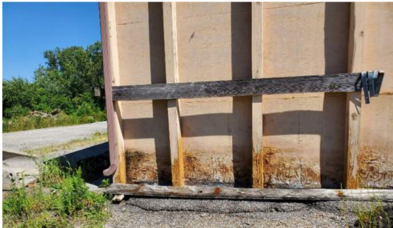
Figure 18. Salt Deterioration on Siding and Poles
