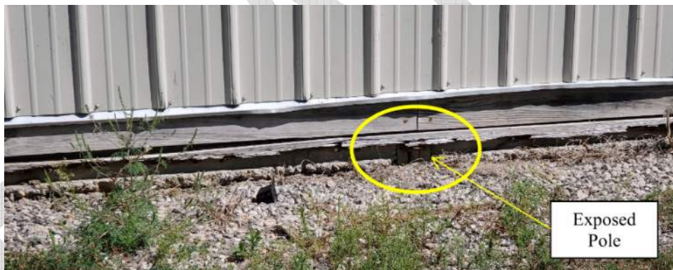
Figure 23. Out-Building 4 Rotting Base Board with Exposed Pole
