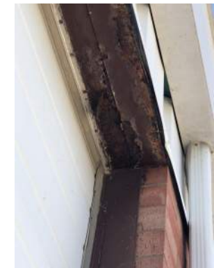
⑦ SCRAPE, PRIME, AND PAINT EXISTING STEEL LINTELS
