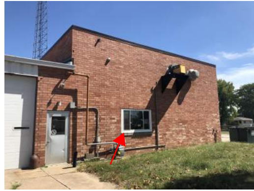
④ REPLACE SEALANT AROUND WINDOW
