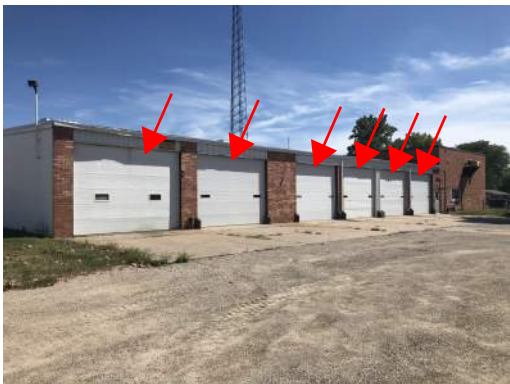
⑦ SCRAPE, PRIME, AND PAINT EXISTING STEEL LINTELS
