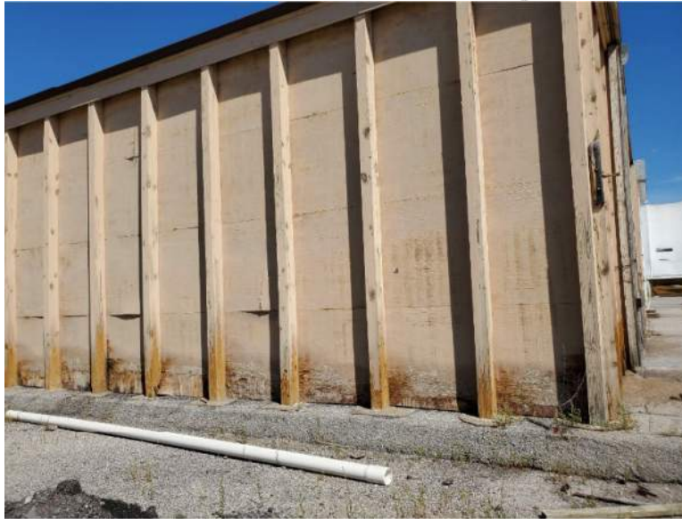
Figure 16. Cracking/Bowing Siding
