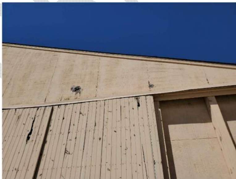
Figure 17. Cracked/Damaged Siding and Door
