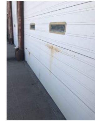
⑩ REPLACE RUSTED OVERHEAD SECTIONAL DOOR
