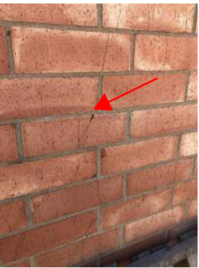
③ REPLACE CRACKED OR SPALLED BRICK
