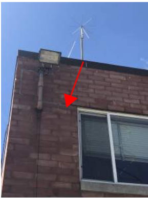
③ REPLACE CRACKED OR SPALLED BRICK
