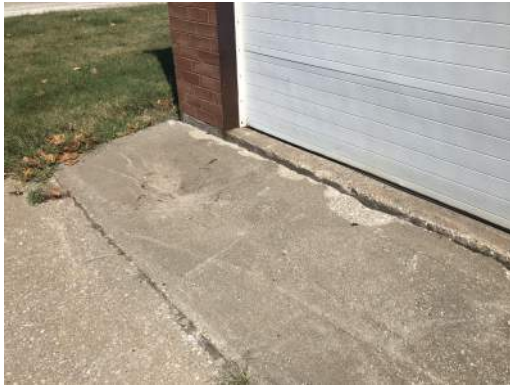
① REPLACE CRACKED AND SETTLED CONCRETE
