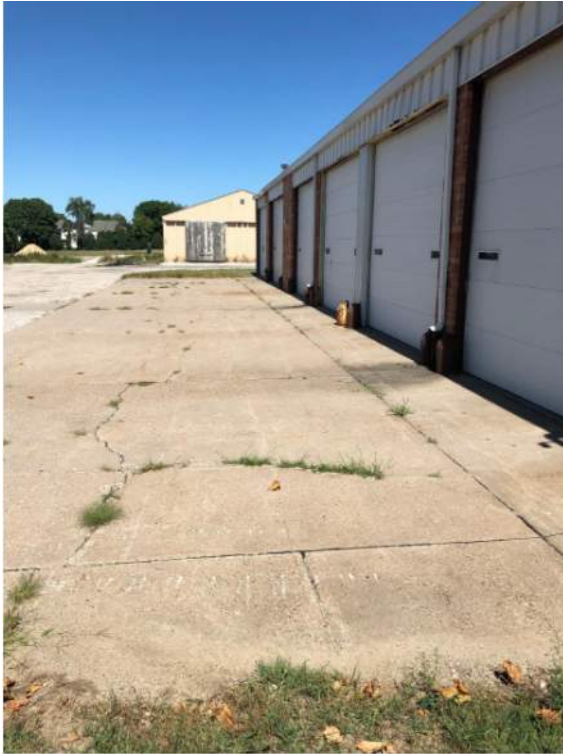
Picture 5: Cracked concrete west of main building. Looking north.
