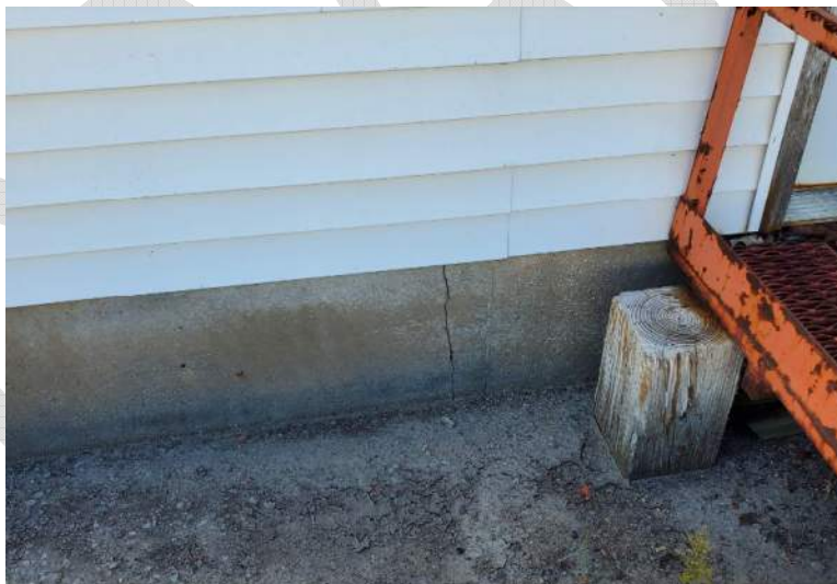
Figure 14. Out-Building 2 Foundation Cracking
