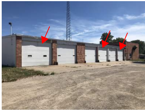
⑩ REPLACE RUSTED OVERHEAD SECTIONAL DOOR
