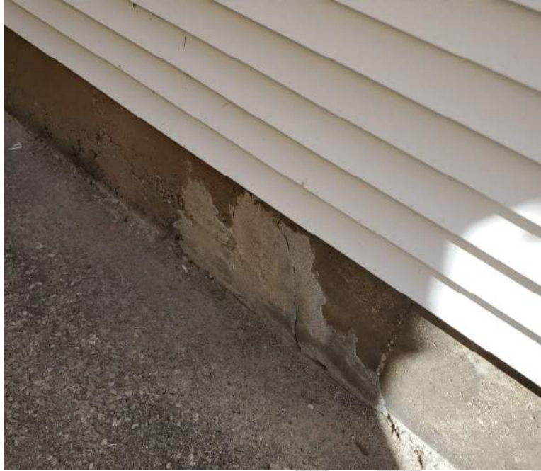
Figure 15. Out-Building 2 Foundation Cracking
