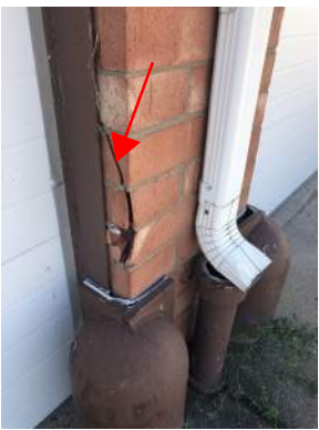
③ REPLACE CRACKED OR SPALLED BRICK
