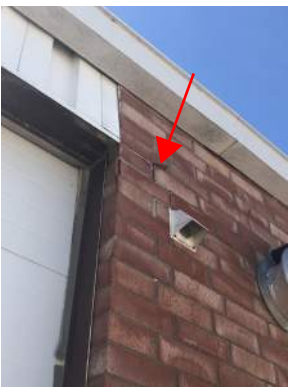
③ REPLACE CRACKED OR SPALLED BRICK
