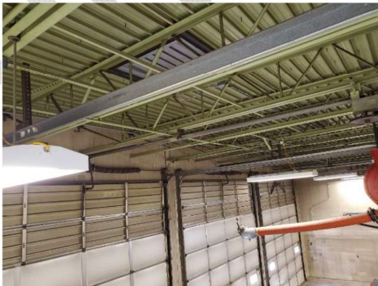
Figure 6. Metal Bar Joists and Roof Decking
