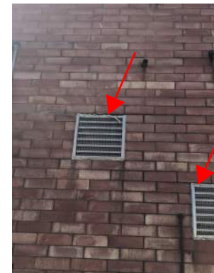
⑥ REPLACE SEALANT AROUND LOUVERS
