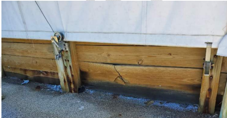
Figure 11. Out-Building 1 Broken Wall Plank
