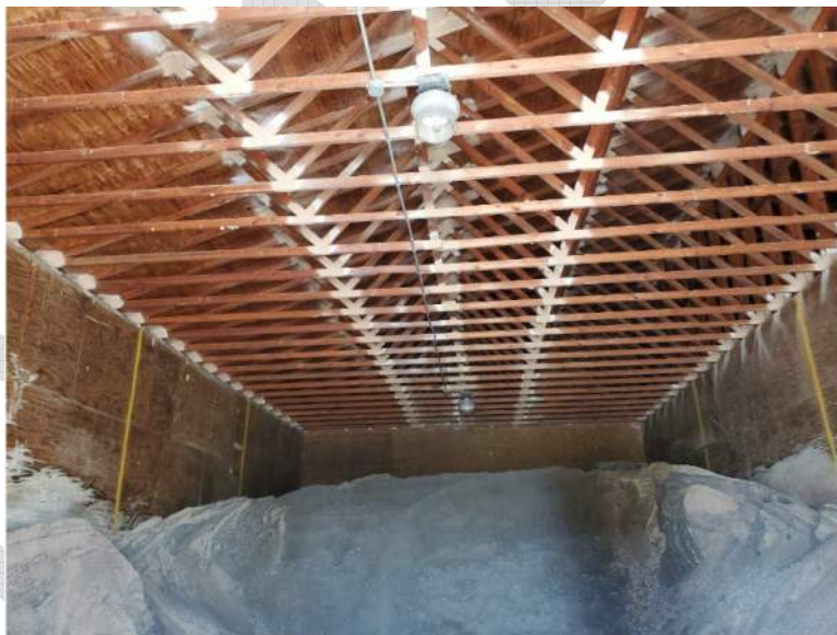
Figure 19. Out-Building 3 Interior Framing
