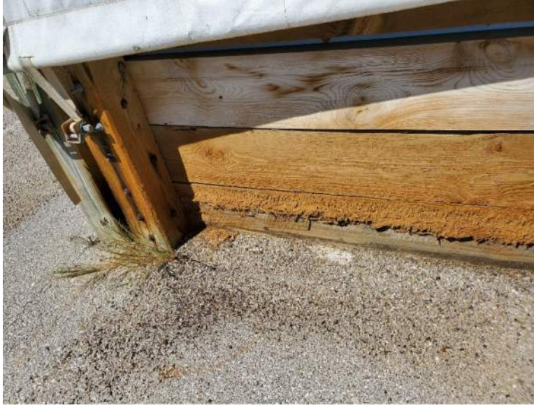
Figure 12. Out-Building 1 Plank Deterioration
