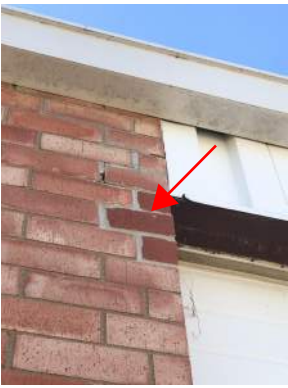
③ REPLACE CRACKED OR SPALLED BRICK
