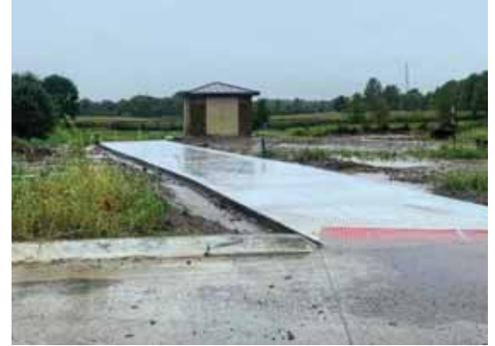
View of new Lift Station and Westside Trail at the Intersection Redwood Dr and Ginkgo Ln
