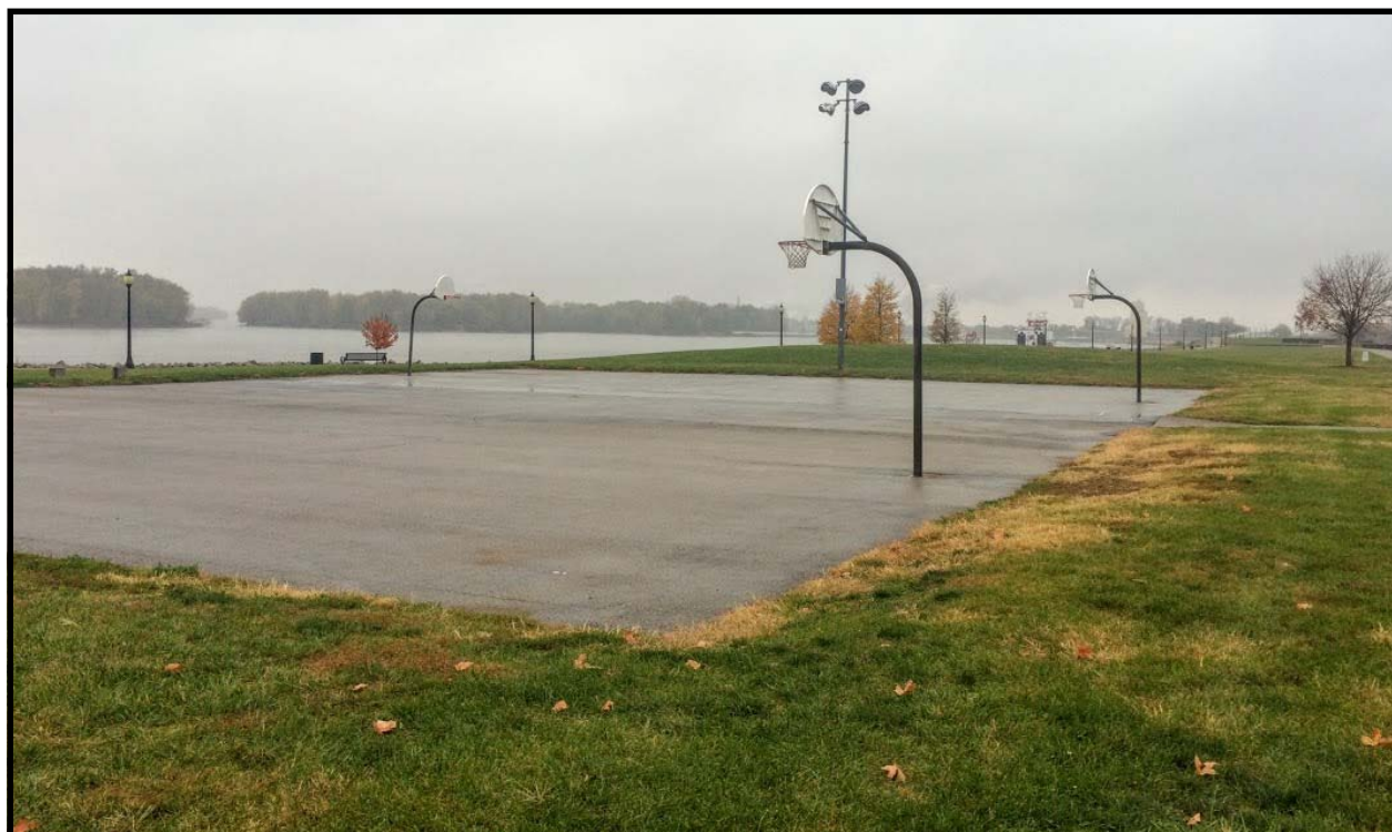
Existing Basketball Court
