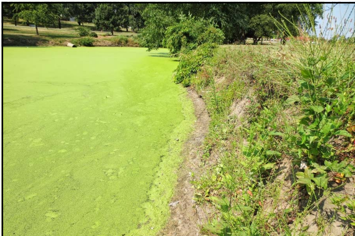
Erosion at the Weed Park Lagoon
