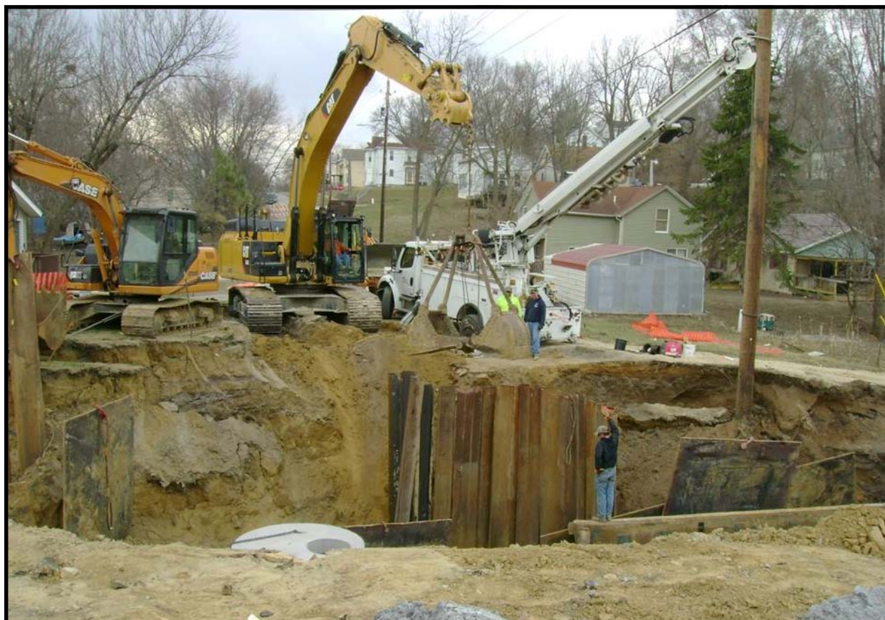
West Hill Sewer Separation Project
