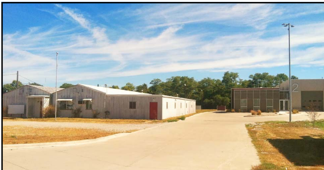
Old Armory Build and Fire Station Number 2
