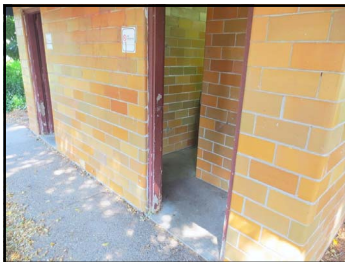
Current Weed Park Restroom Facilities
