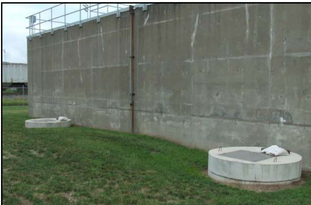
Figure X: Existing Quad Valves
