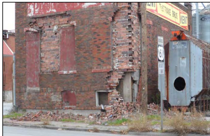
Southwest Corner Showing Damage to Puritan Ice Building
